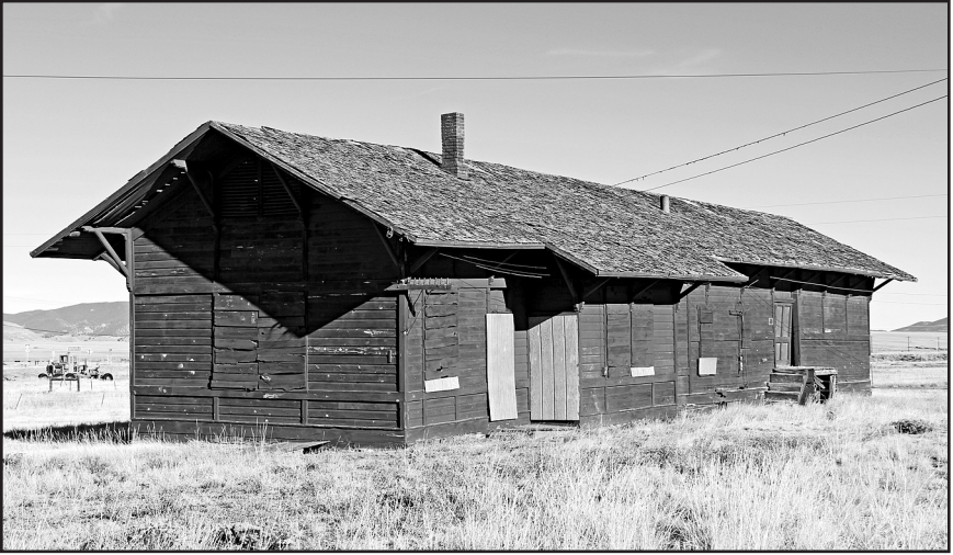
The Colorado Midland depot still stands at Hartsel, Colorado, on November 29, 2011. – Photo © 2011 Dave Schaaf.
